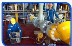
General problems associated with bolted joints are incorrect joint assembly, improper tightening methods, ineffective flange tagging systems and lack of formal flange control / management system.
